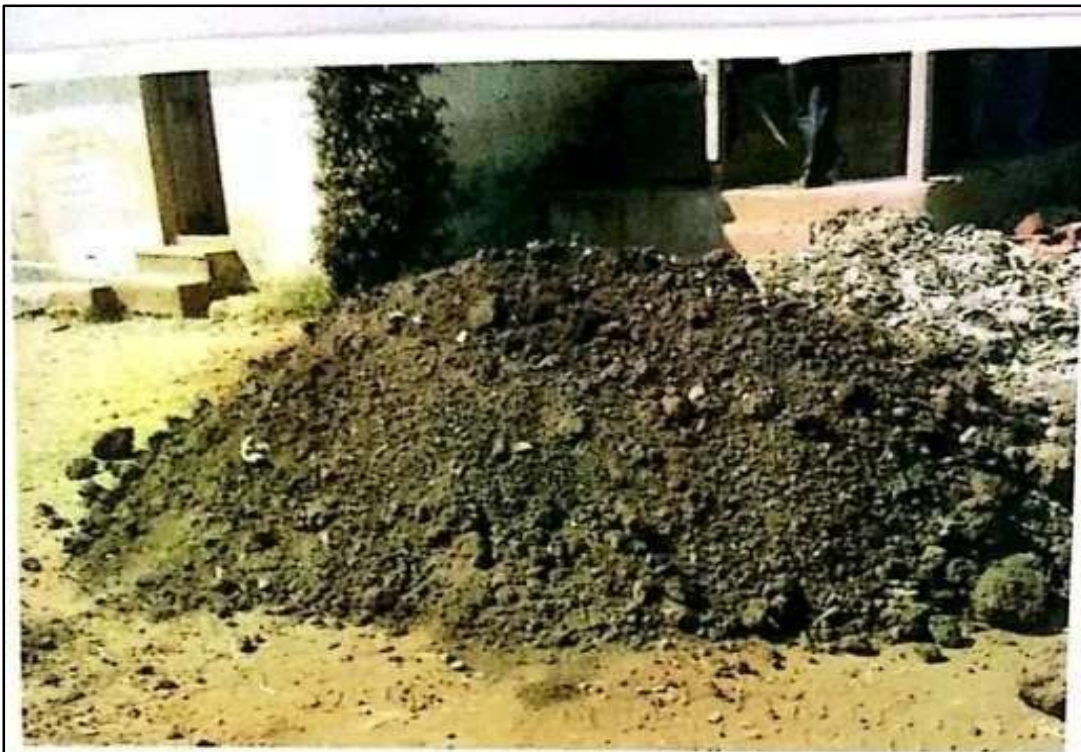
Filling or laying of Soil
